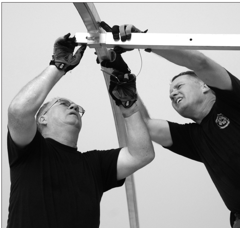
Below: Tech. Sgt. Gary Risen and Lt. Col. Bill Adkisson of the 123rd Medical Group connect beams used in the support structure of EMEDS facilities.
