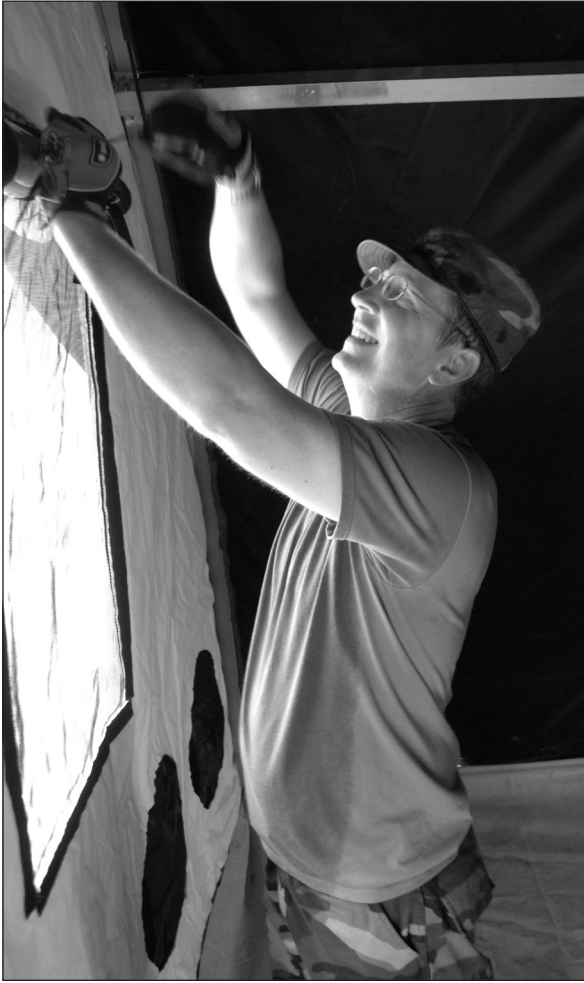
Above: Tech. Sgt. Mark Duke, a health services manager, secures windows that are being installed in an EMEDS facility.
